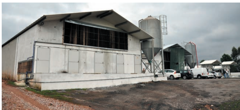
NORLAP. Vista exterior de las naves.
